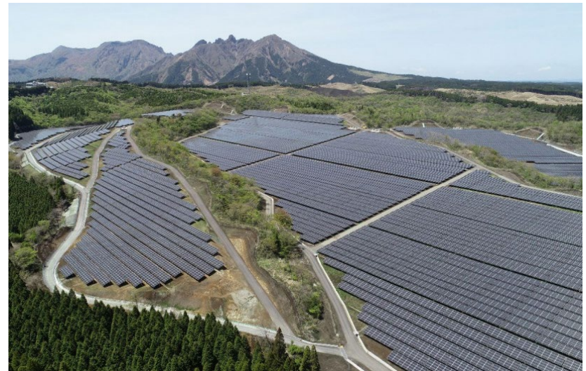
JRE Aso Takamori Solar Power Plant Project
